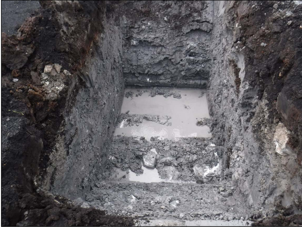
Photo 3 Trial Pit TP/T13
