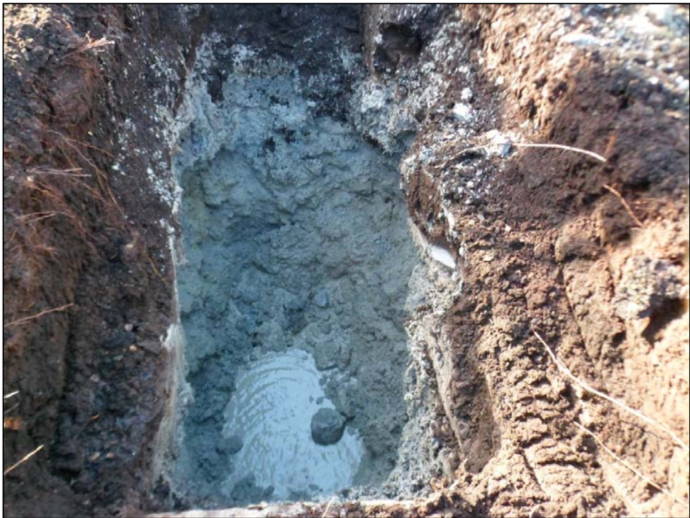
Photo 4 Trial pit TP3
