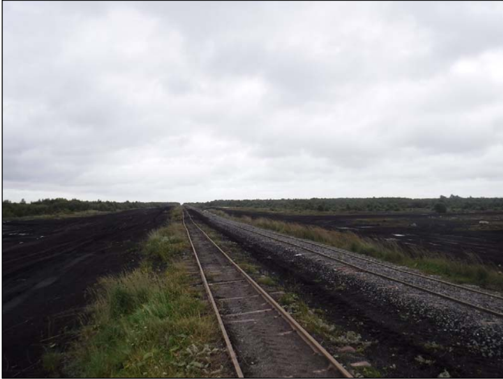
Photo 5 Example of Bord na Móna existing rail lines on site (close to turbine T17 looking in a north-eastern direction)
