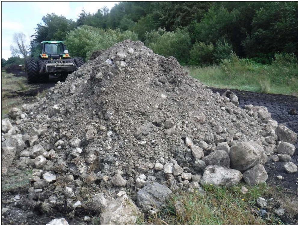
Photo 8 Excavated arisings from trial pit TP/CSH2
