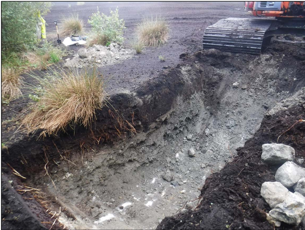
Photo 4 Trial pit TP/T17
