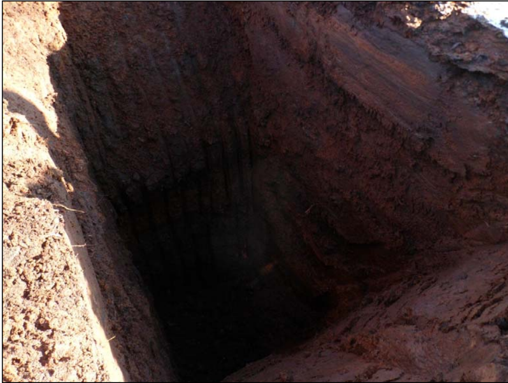
Photo 13 Trial pit TP11
