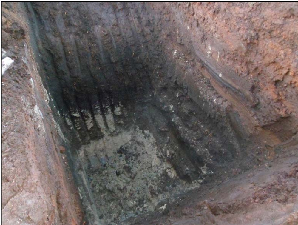
Photo 12 Trial pit TP10
