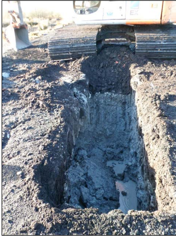
Photo 1 Trial pit TP1
