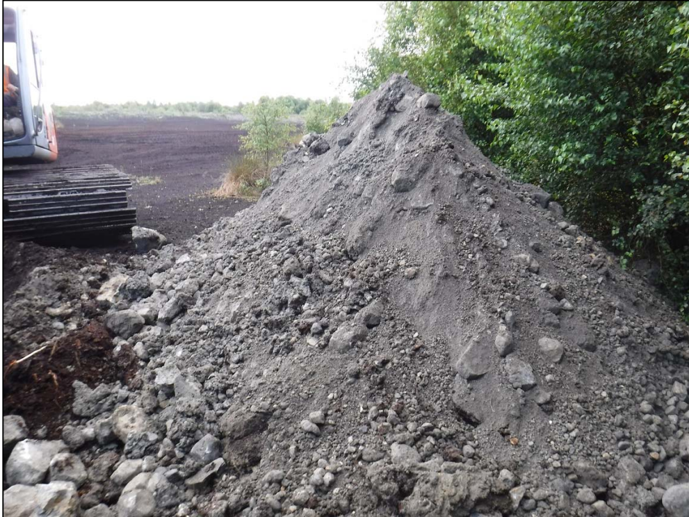
Photo 5 Excavated arisings from trial pit TP/T17
