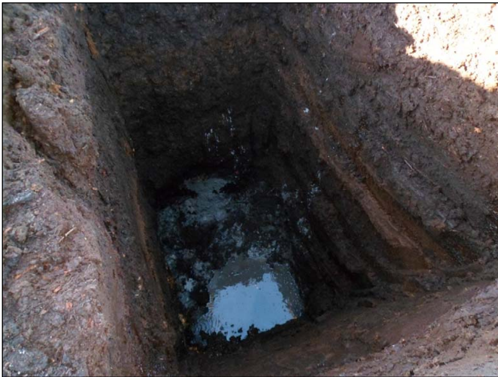
Photo 14 Trial pit TP12
