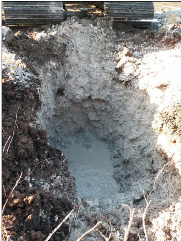
Photo 2 Trial pit TP2
