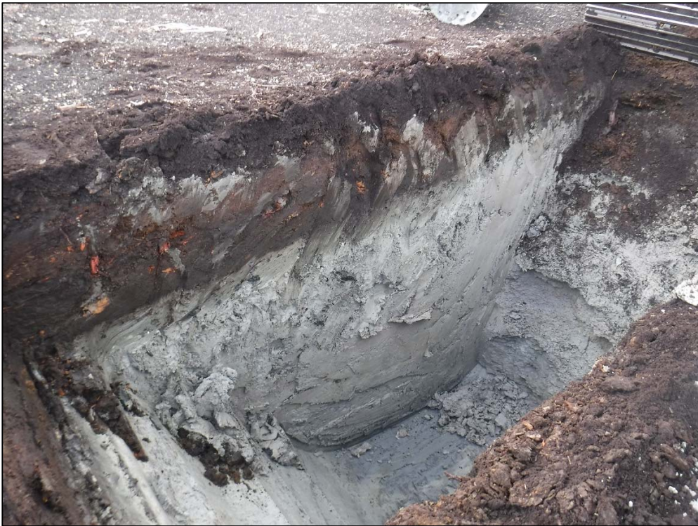
Photo 14 Trial pit BP3/TP2
