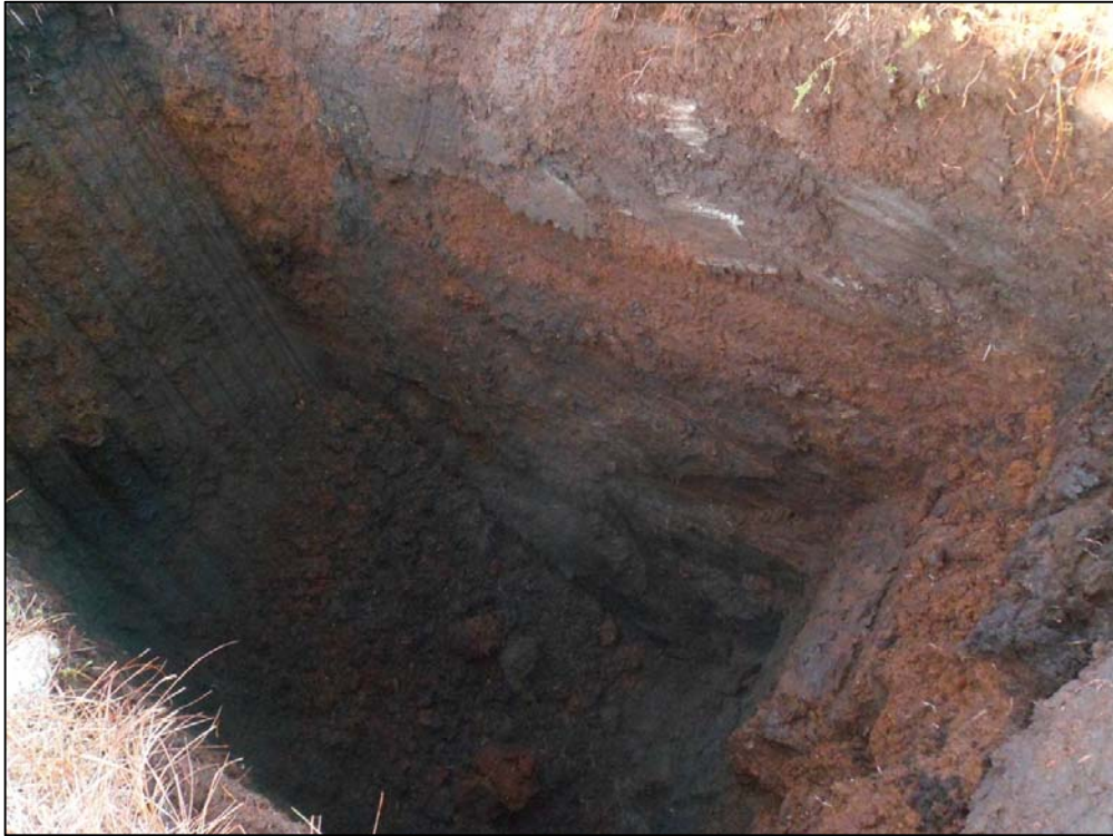
Photo 11 Trial pit TP9
